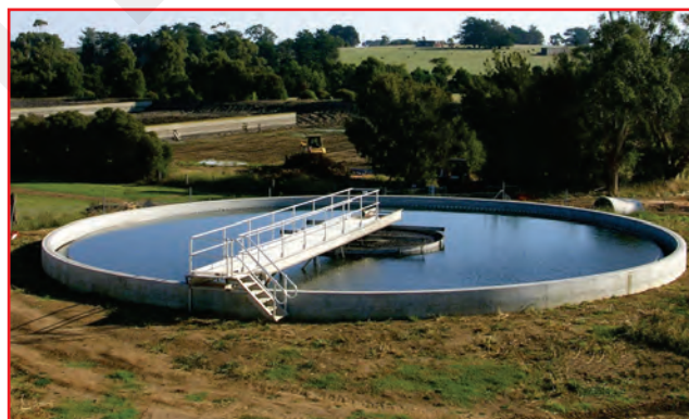
Sedimentation of tank
